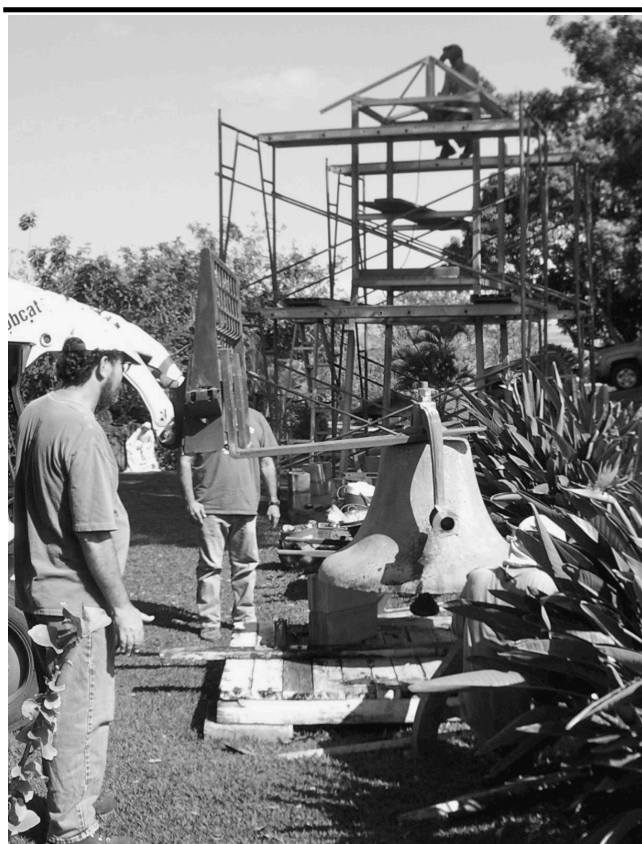
The bell is lifted off its stand and onto temporary blocks. In the background, welding continues on the top portion of the tower.
